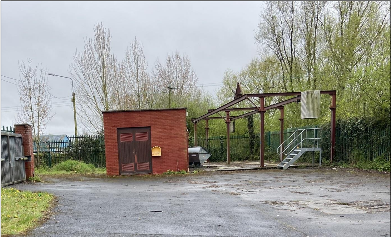
Figure 2-2 – View of existing Kilkenny Road Pump Station (Photograph from AtkinsRéalis site visit)
